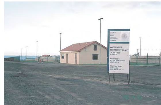
General view of the control and laboratory building
