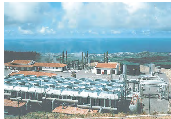
General view of the Ribeira Grande Geothermal Plant Foreground: the condenser yard
