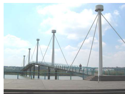
Topo: A ponte acabada. Top: The finished bridge.
