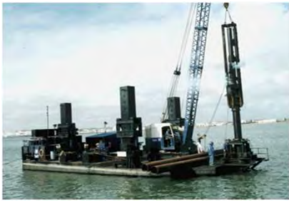
Jack-up platform "Valeira" Marine pile driving
