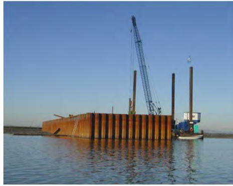
Coferdam (sheet piling) HDD Works for Sines-Setúbal Pipeline
