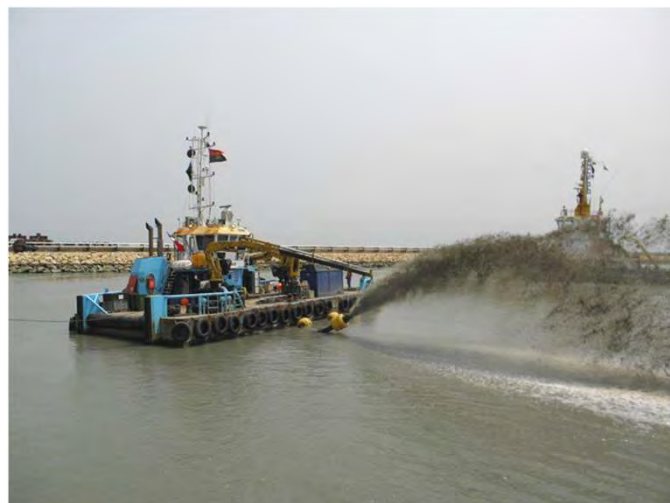
Dredging with DOP pump
