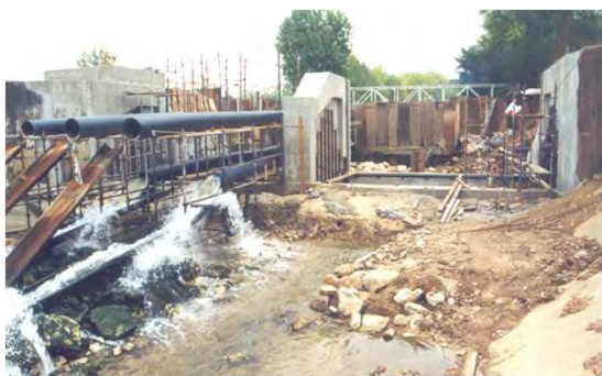
Inflatable weir at Arrabalde: river to flow only in the lower tubes, during the execution of work
