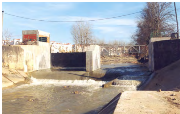
Inflatable at Arrabalde: view downstream of the two spans, cofferdam and house to electrical controls
