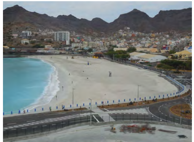
Laginha Beach after completion of sand filling
