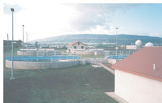
General view of the WWTP. Background: the clarifier tanks
