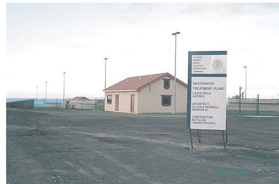
General view of the control and laboratory building
