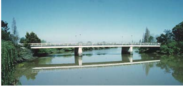
The "Vala Nova" Bridge The first pre-stressed concrete bridge in Portugal Built by SETH in 1954
