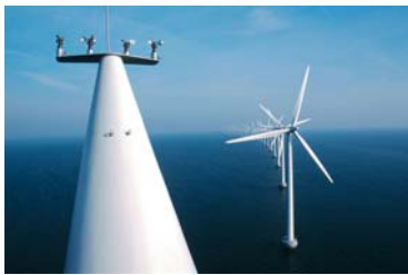
Offshore Wind Turbines Denmark
