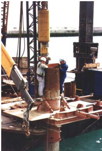
Special foundations: marine pile driving (tubular and sheet). SETH is the undisputed leader of this sector in Portugal
