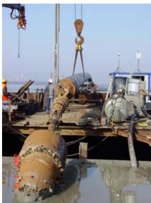
Sines-Setúbal Gas Pipeline HDD Works (Sado River)
