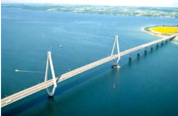
Farøbroen Bridge Denmark
