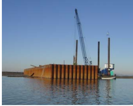
Coferdam (sheet piling) HDD Works for Sines-Setúbal Pipeline
