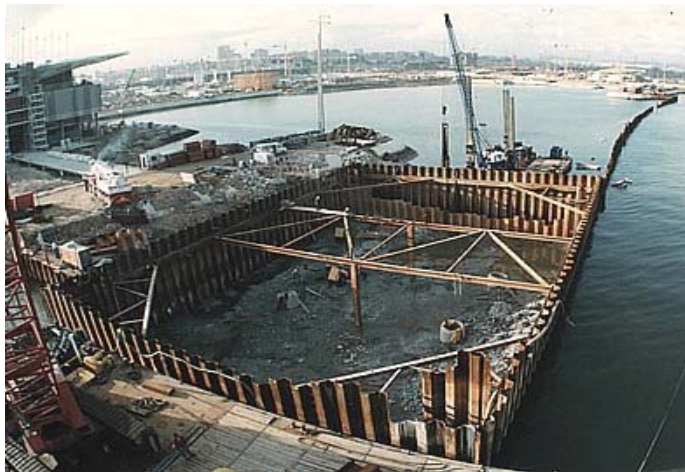
EXPO '98 Olivais Dock Lock cofferdam
