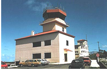
U.S. Navy Control Tower / RAPCON Lajes Field, Azores
