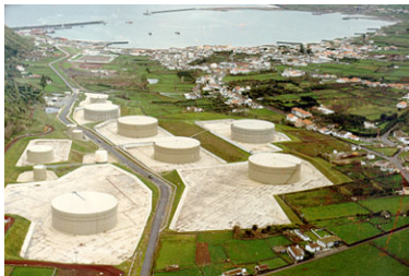
U.S. Navy Repair of POL tanks Lajes Field, Azores
