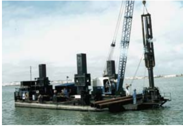
Jack-up platform "Valeira" Marine pile driving
