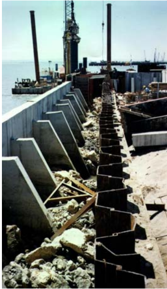
Sheet-pile curtain wall
