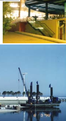
EXPO '98 Olivais Dock Amphitheater Pile driving
