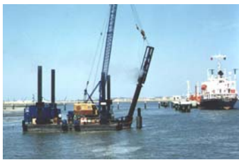
Petrogal - Aveiro Marine pile driving
